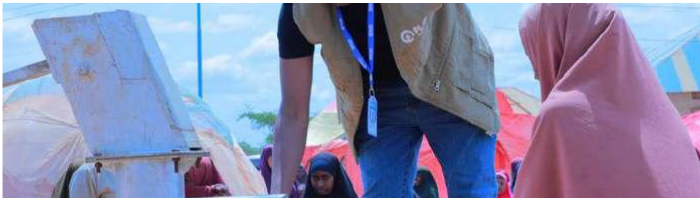
Borehole and handpump water point | Photo: READO
